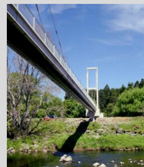
Award Winning New Plymouth Water Supply Cable Stay Bridges
