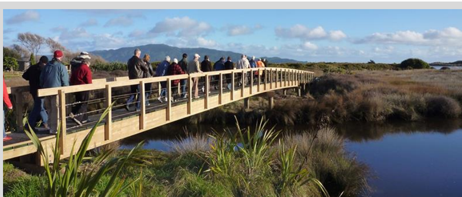
Waikanae Estuary Bridge
